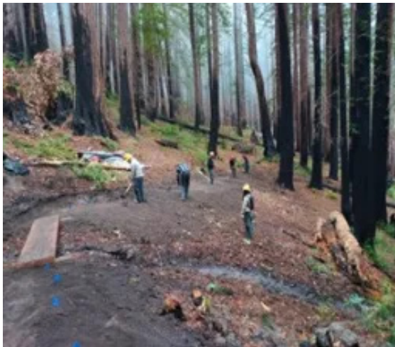
Crew Reconstructing Trail
