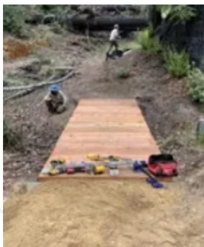
Foot Bridge - Skyline to the Sea trail
